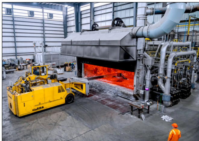
Figure 2. A semi-automatic machine skims the surface of the melting furnace.
